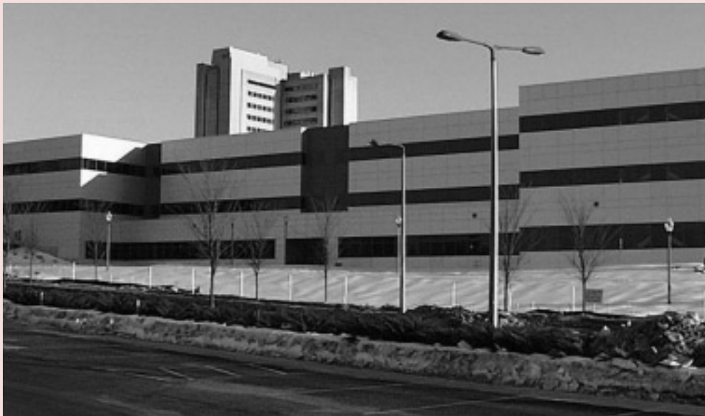
Work proceeds apace on the new Computer Science facilities, which are steadily nearing completion.
